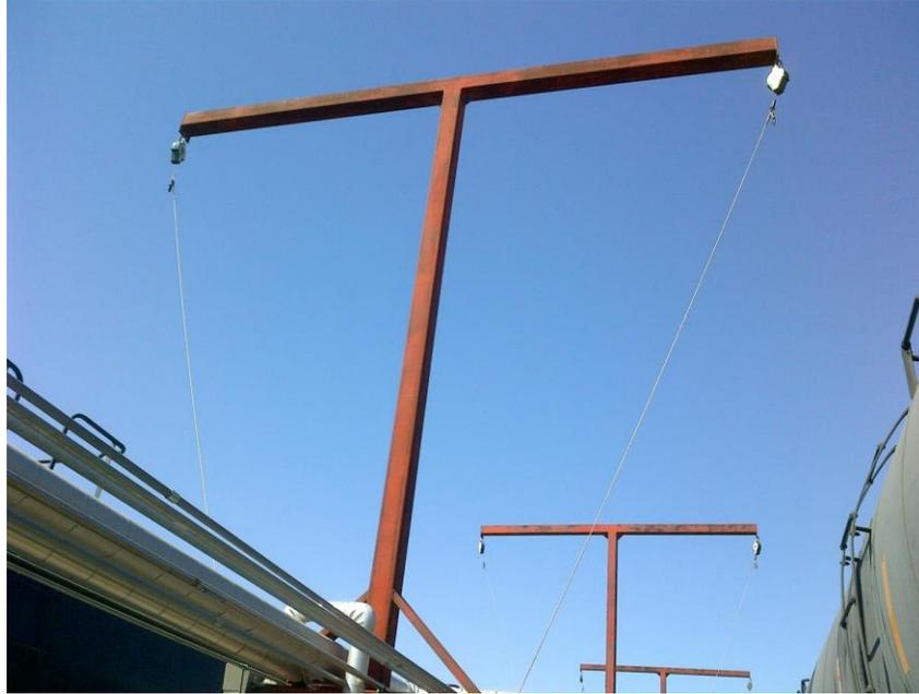
If a fall protection system is not available at a consignee, a lanyard and harness might be attachable to the trailer. **CAUTION:** The trailer anchor point must be rated for 5000 pounds of static force. Below is an unacceptable method of attaching a lanyard and harness to a trailer.
